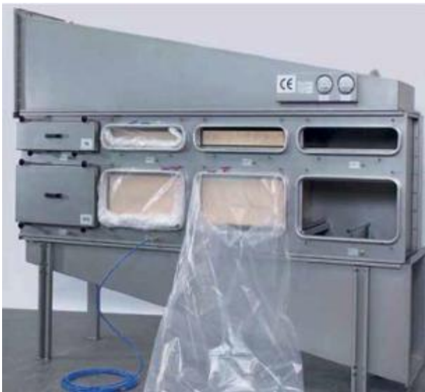
Fig 8a and b. Modern Multi Bank “Safe Change” Filter Housings With Pre-Filters (Top) and HEPA Filter arrangement at the bottom.
