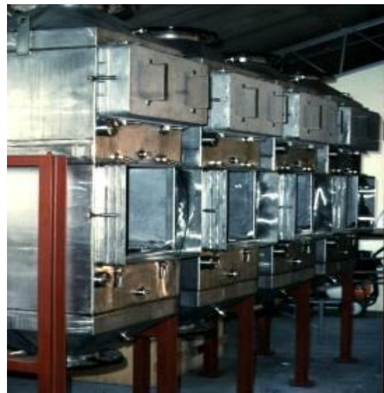
Fig 8a and b. Modern Multi Bank “Safe Change” Filter Housings With Pre-Filters (Top) and HEPA Filter arrangement at the bottom.
