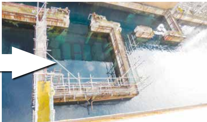
FIGURE 2: Pond walls after clearing
