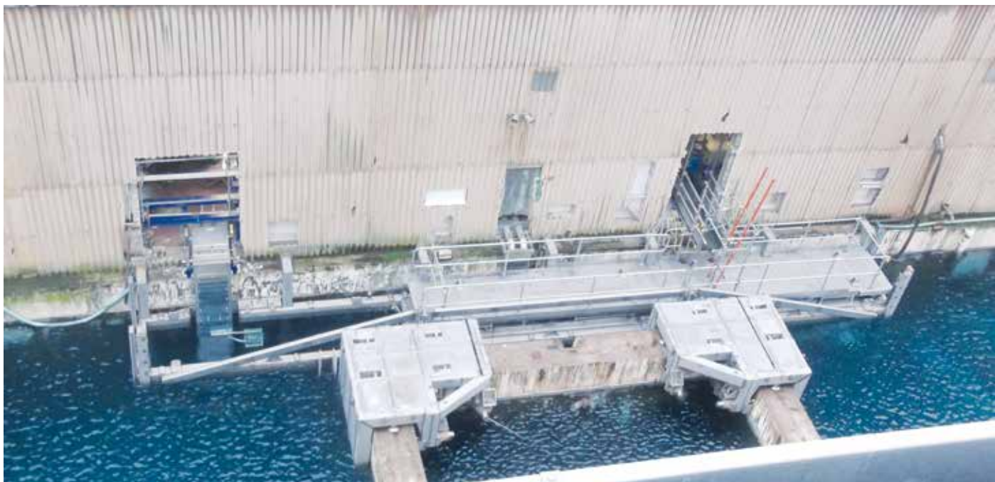
FIGURE 5: Pond platform 2 installed
