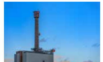
Self Climbing Platform (SCP) Stack Demolition – Sellafield, UK
