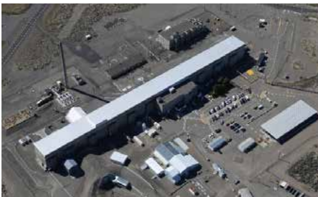
FIGURE 9: T separation plant building, Hanford, under construction (top) and (bottom) operational in the 1950s. This plant – the first operational ‘canyon’ - received its first irradiated fuel in November 1944. (Top photo - public domain. Bottom photo – Gerber 1994).
