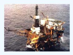
The main workings had to be situated close to the control room and accommodation block, this was to prove fatal to many of the workers on the rig. The cladding was fireproof but was not rated for withstanding an explosive force.
