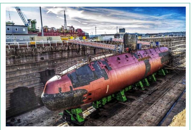
The Submarine Dismantling Project aims to deliver a safe, secure and environmentally responsible solution for dismantling 27 of the UK's defuelled nuclear-powered submarines following their exit from service with the Royal Navy.
